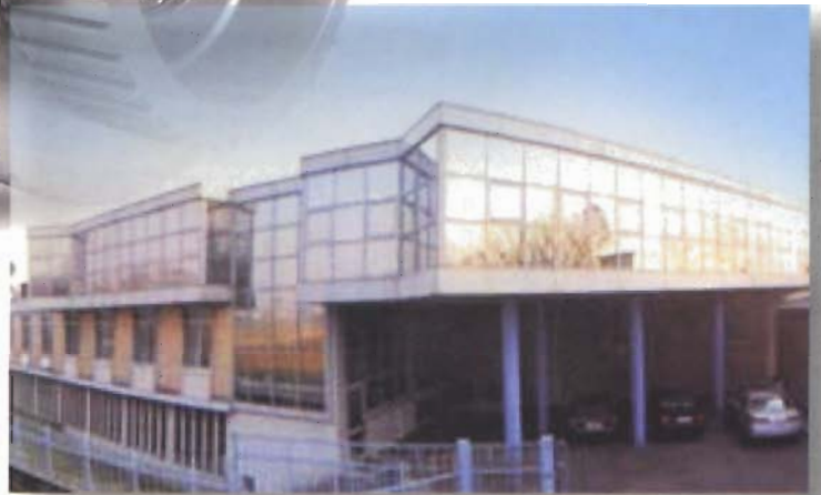
Milan (ITALY) - Production plant for standard and special pulleys.
