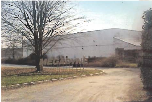
New plant in Mathi (ITALY) Polyurethane endless extruded Megaflex belts production.
