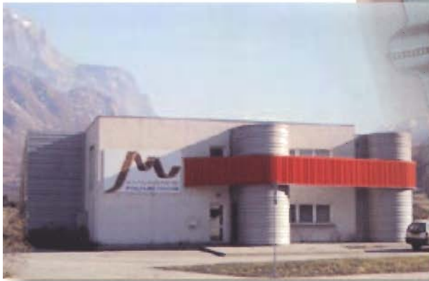
S.te Jean de Maurienne (FRANCE) Polyurethane moulded endless timing belts production.
